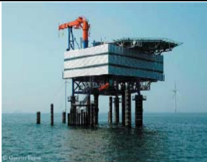
Figure 5.4 Indicative Model of an Offshore Substation at Horns Rev Offshore Wind Farm (Denmark) (1)
