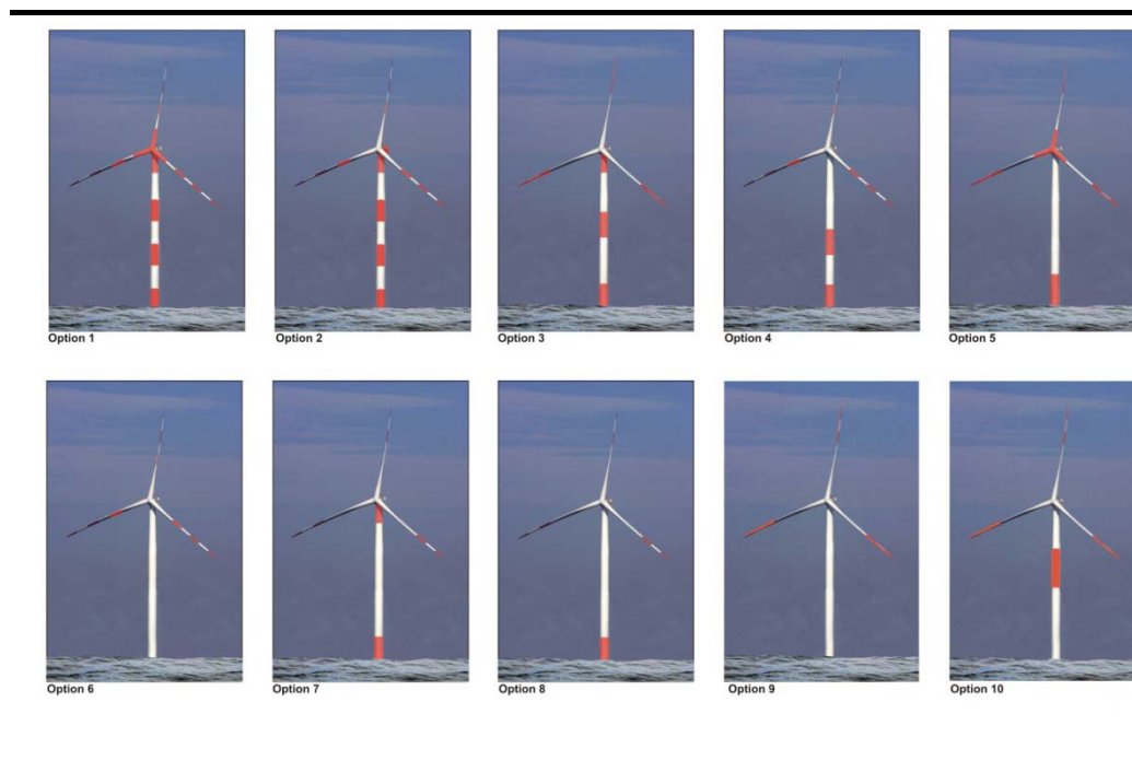
Figure 4.11 Turbine Marking Options
